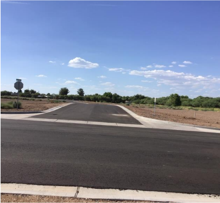
VIEW FROM N HOMESTEAD PARKWAY
