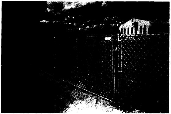
tencing to be chain link with 3 strand barbed wire. Total heighth of fence to equal 7'. Commercial fencing may be 8' according to Section 108 E. Z. b. 2),
