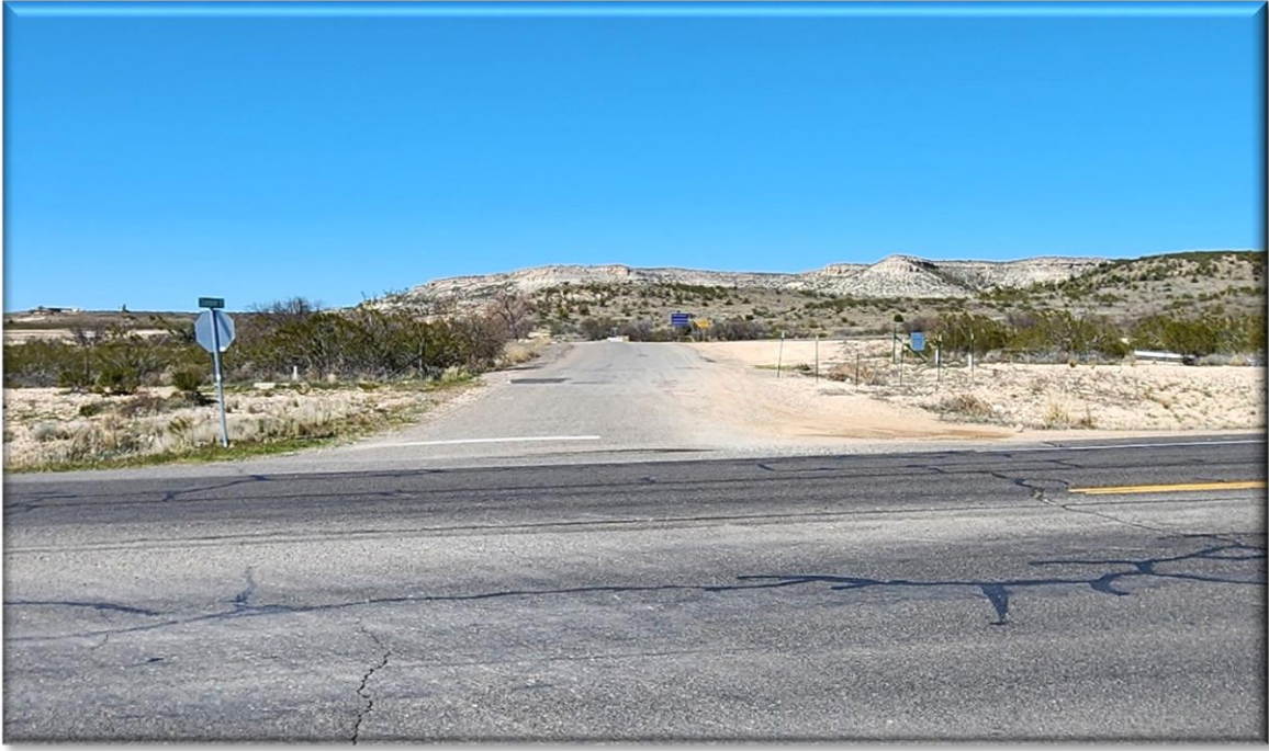
Champion Trail at Highway 260. Note that the asphalt on Champion Trail is only slightly wider than the southbound lane out of the complex. The right turn lane onto Champion Trail off of Highway 260 is dirt with poor drainage.
