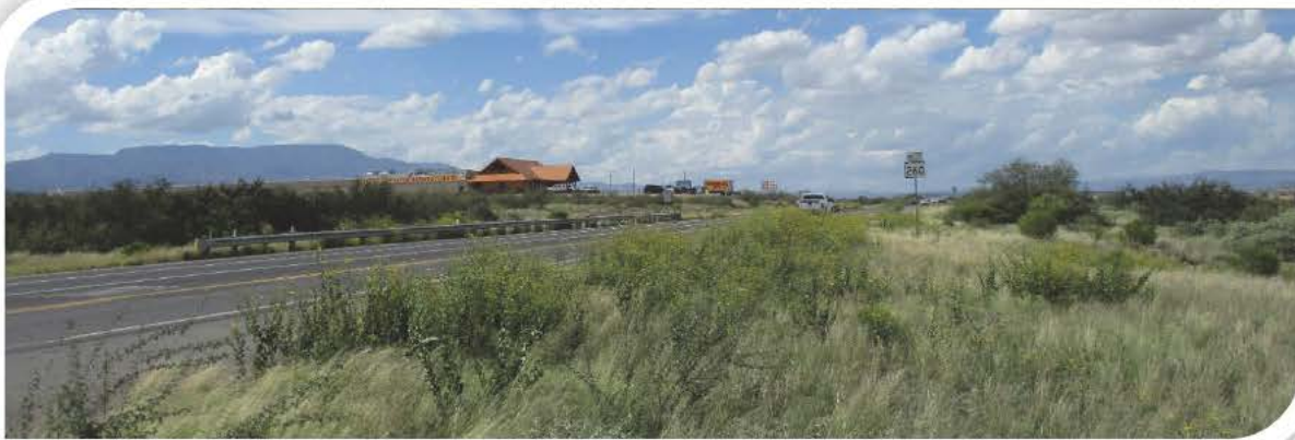
260 Corridor Near The Intersection Of State Route 260 & Cherry Creek Road Photo Courtesy Of The Town Of Camp Verde Community Development Department
