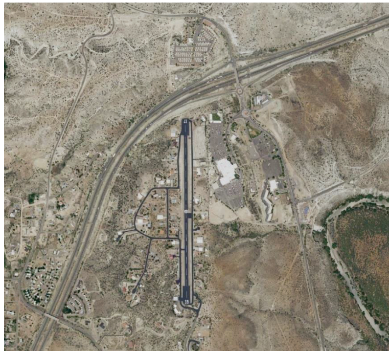
Aerial Imagery Of A Portion Of The Pecan Lane Character Area Photo Courtesy Of Yavapai County GIS
