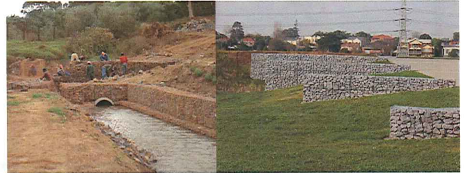
Gabions in use
