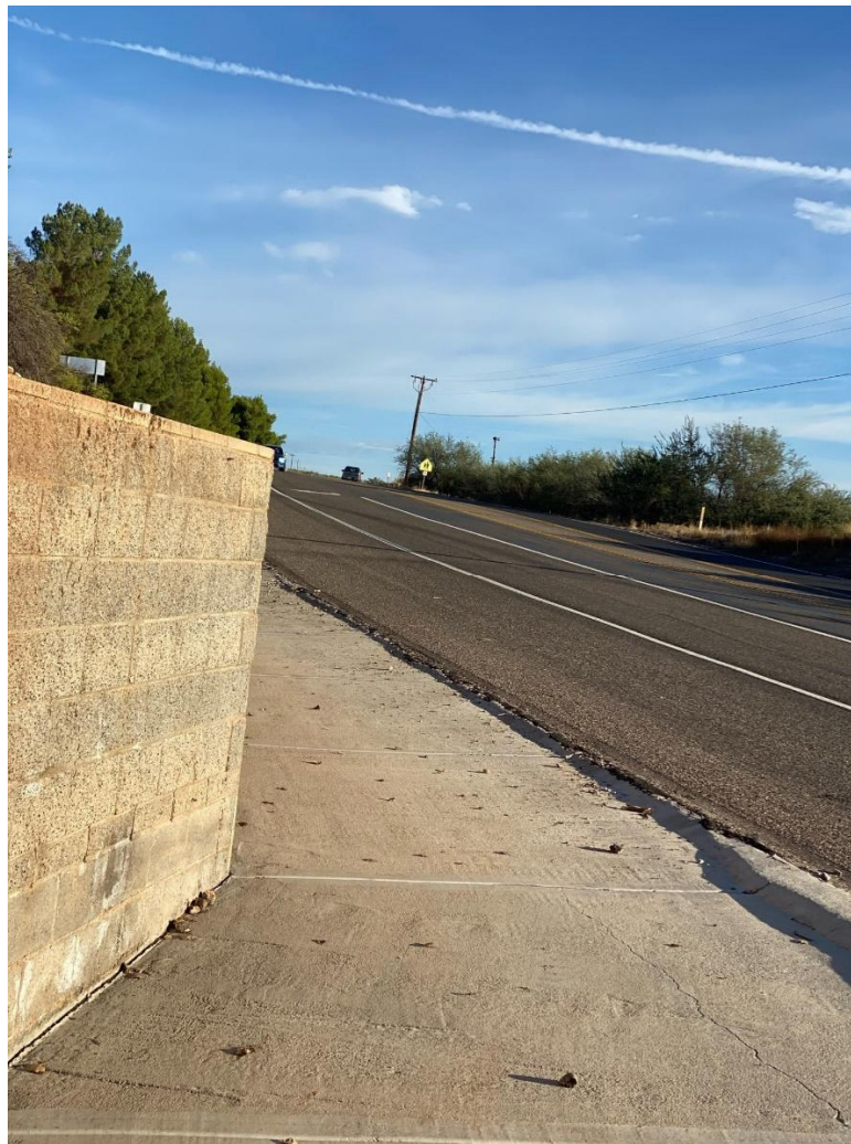
Figure 3. Sight-Distance at North Montezuma Castle Hwy & Camp Lincoln Rd Looking Northbound
