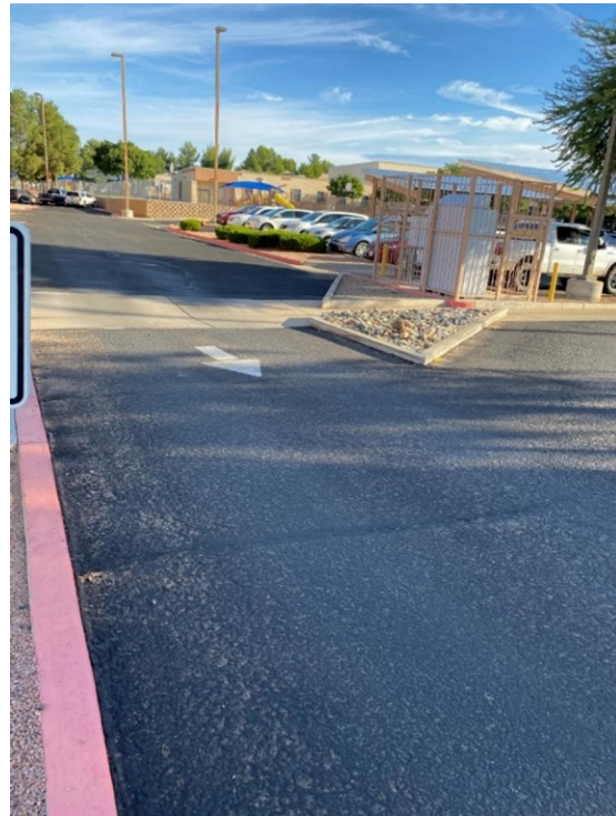
Figure 10. Egress Traffic at Driveway
