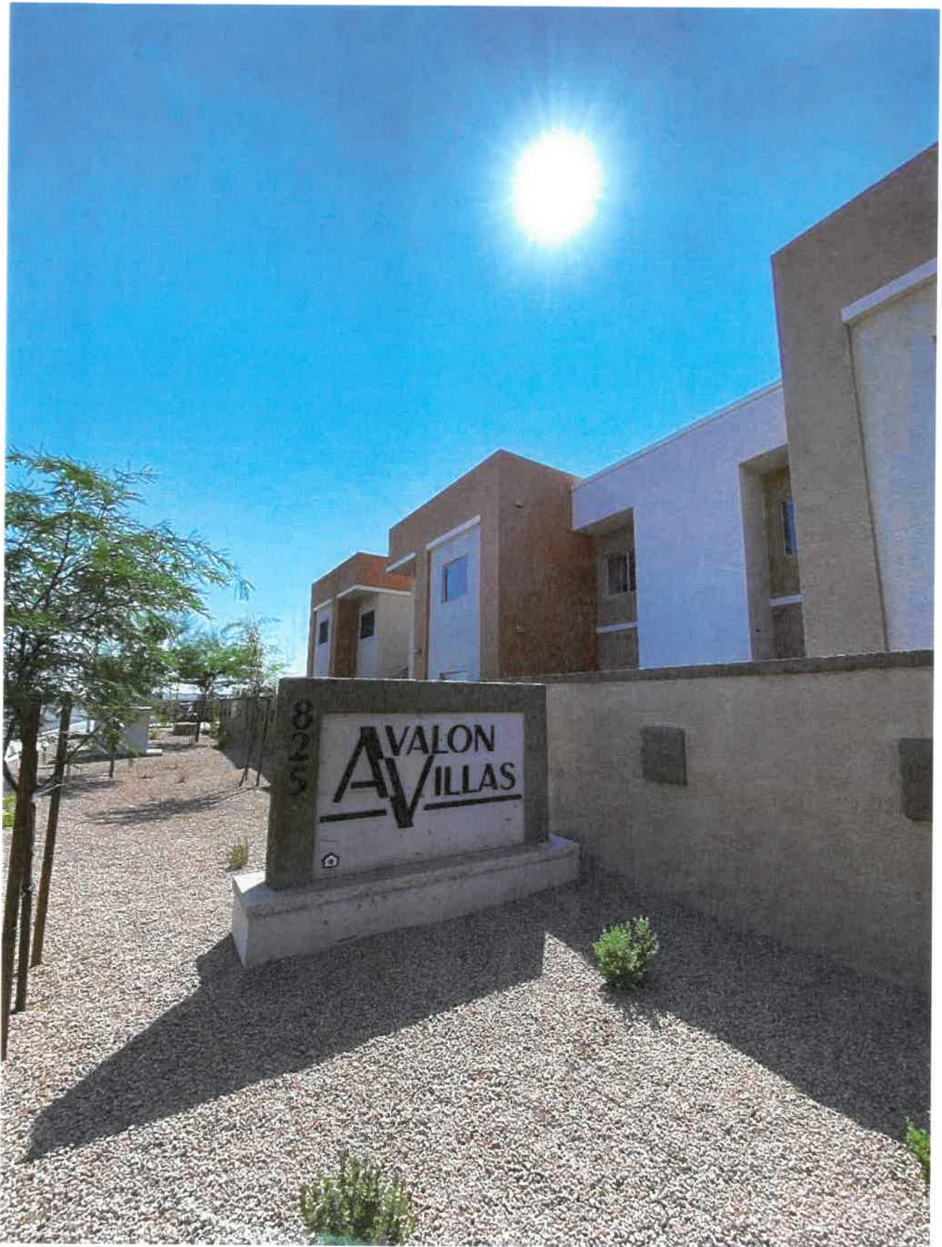
Figure 1. Typical Exterior of Townhome/Flats
