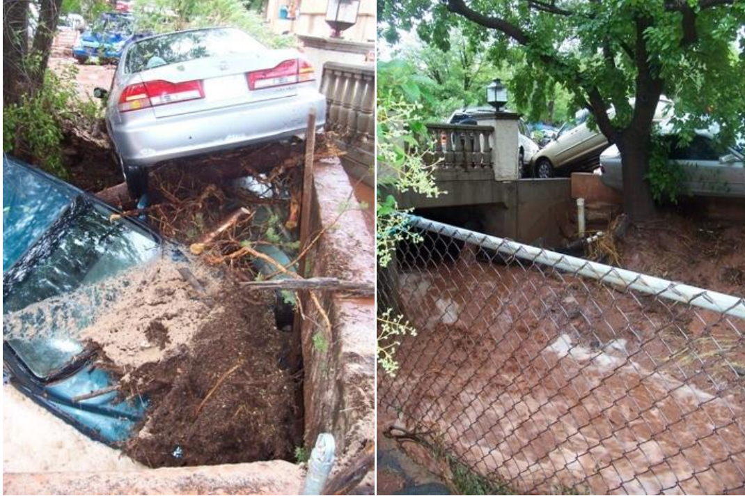
2010 Sedona Flood Damages
